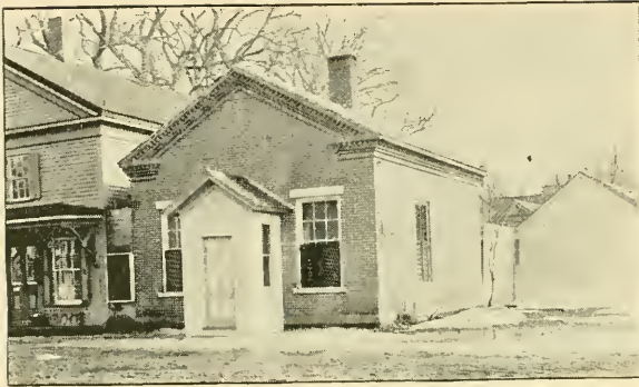
Town Building, Plymouth Center.
